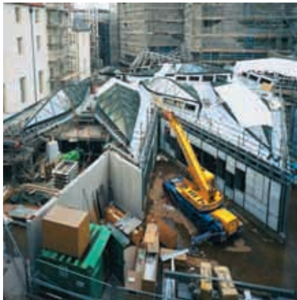
Foyer roof lights
