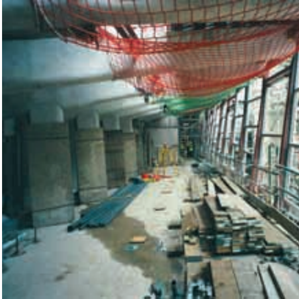
Construction of glazed walkway providing access to Chamber for MSPs
