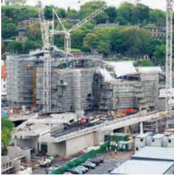
Landscaping works viewed from Salisbury Crags
