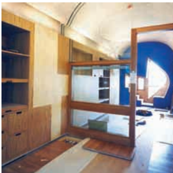
Internal fit out of MSPs' offices
