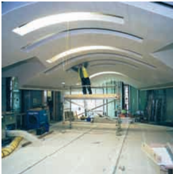
Construction of Committee Room ceilings
