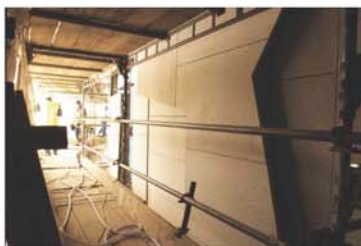
Stone trigger panel can only be installed when blast windows are complete.
