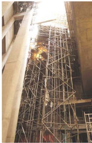
Tower scaffolding preventing current access to lightwell.
