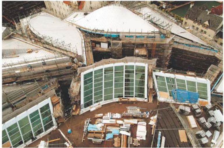
Aerial view of lightwell highlighting access restrictions from adjacent structures.
