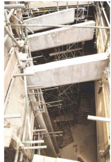
View from link bridge depicting access restrictions into lightwell.
