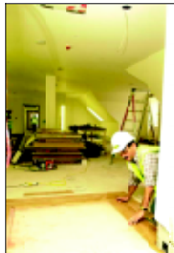
Installation of timber floors on the fourth floor in Queensberry House.
