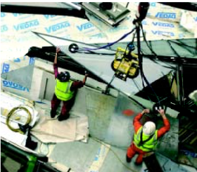
Final pieces of glazing being installed to Lobby rooflight.
