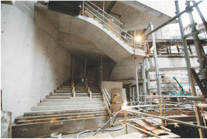
Progress continues on the public stair.
