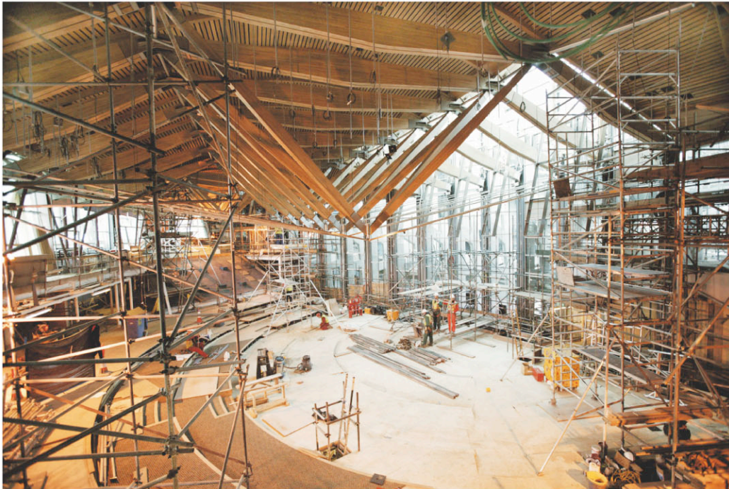
The dramatic oak ceiling spans 60 metres in length and 30 metres in width.
