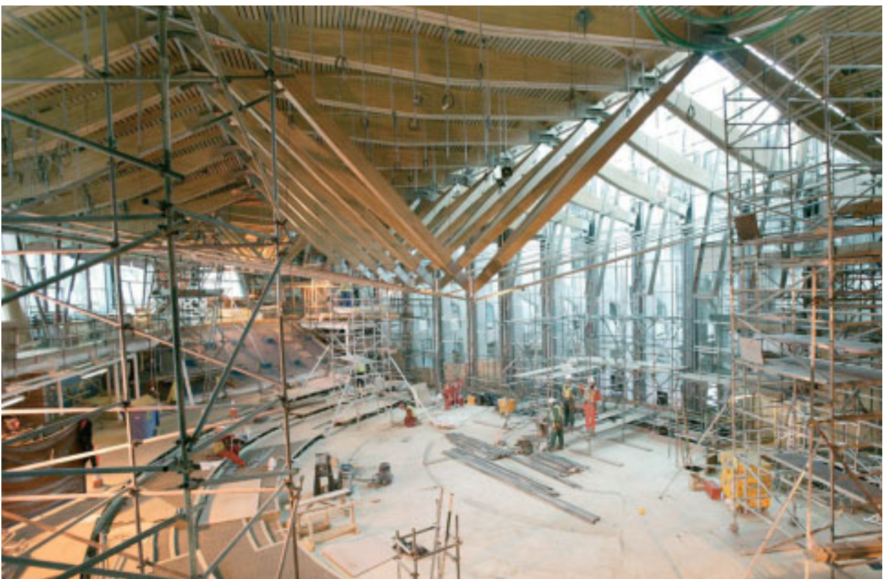
Debating Chamber ceiling beams
