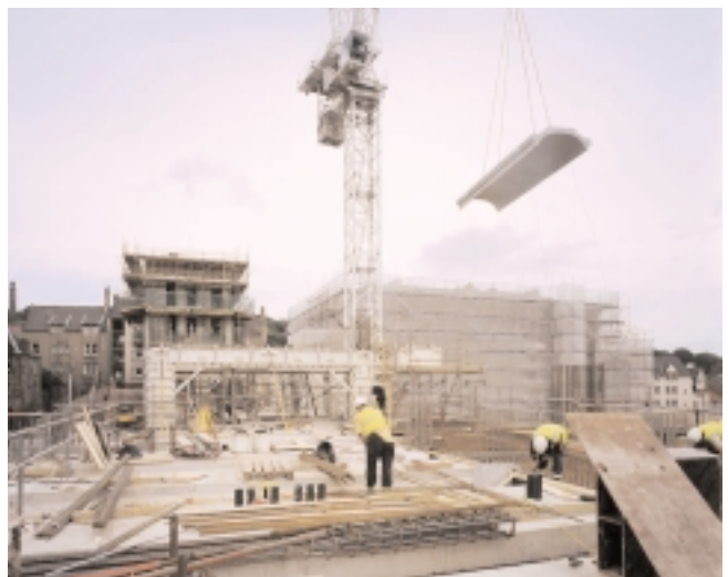
Pre-cast concrete ceiling unit lowered into place
