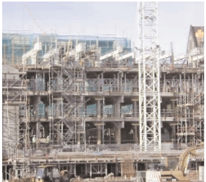
Work progressing on MSP building - September 2000
