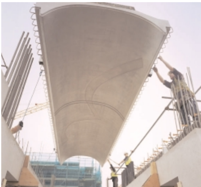
Detail of pre-cast concrete ceiling unit
