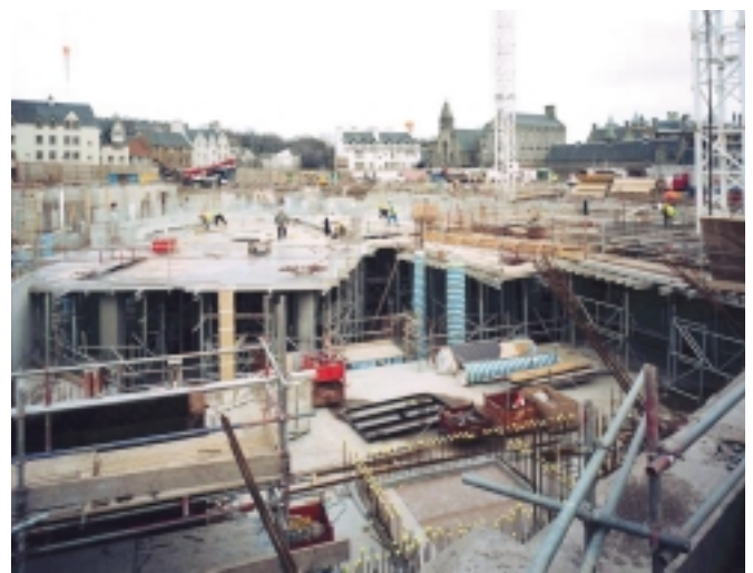
Construction progressing on Debating Chamber and Committee Towers
