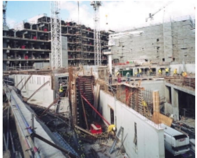
Construction work in progress
