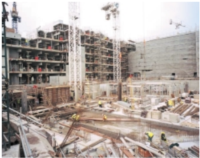
The MSP building reached its fullest height in January
