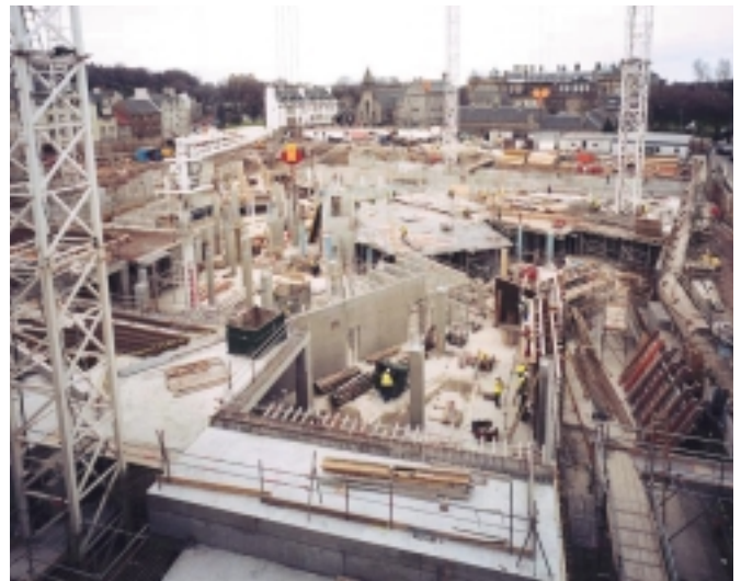
Construction of Debating Chamber and Committee Towers commenced in October 2000
