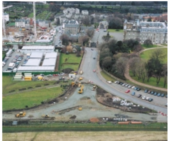
Work underway on the upgrading of Queen's Drive
