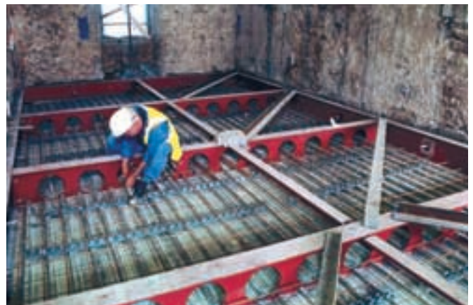
Work under way on replacing floors within Queensberry House
