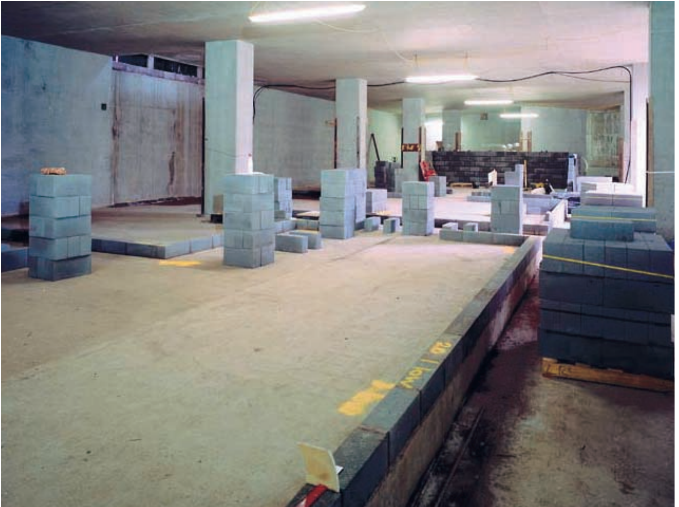
Work under way in the east basement
