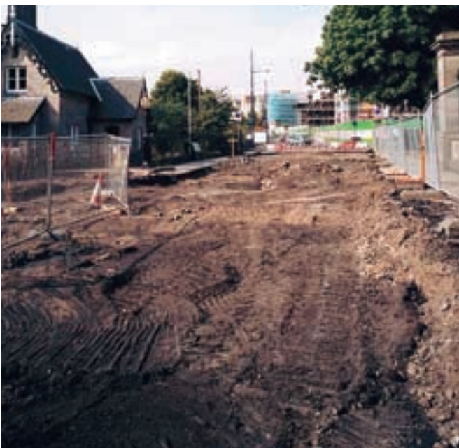
Upgrading of existing road structure
