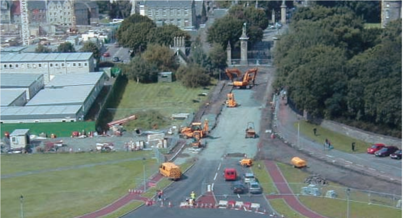
Upgrading of Queen's Drive Spur
