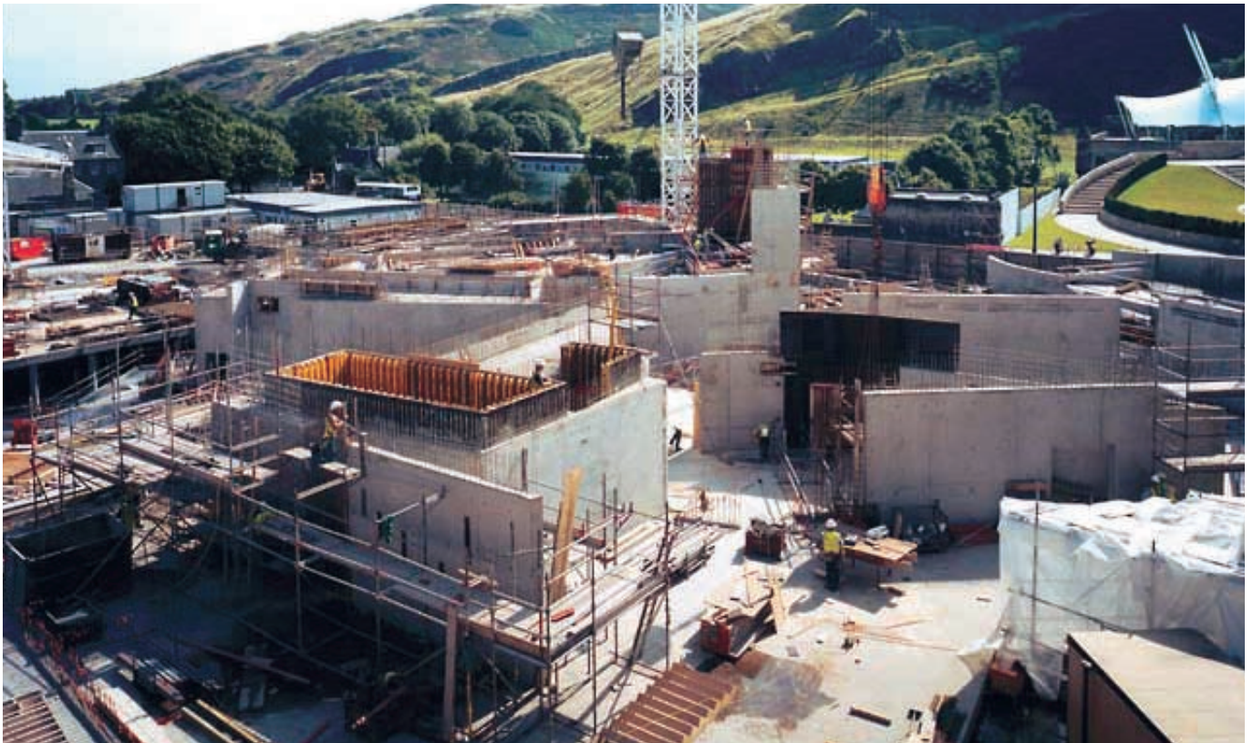
Construction of Committee Towers
