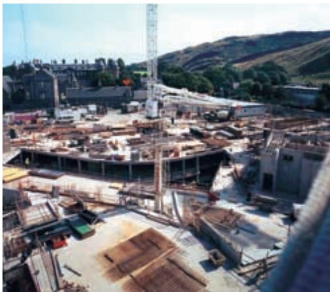
Construction of Debating Chamber
