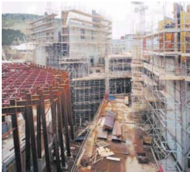
Construction of Chamber and Committee Towers
