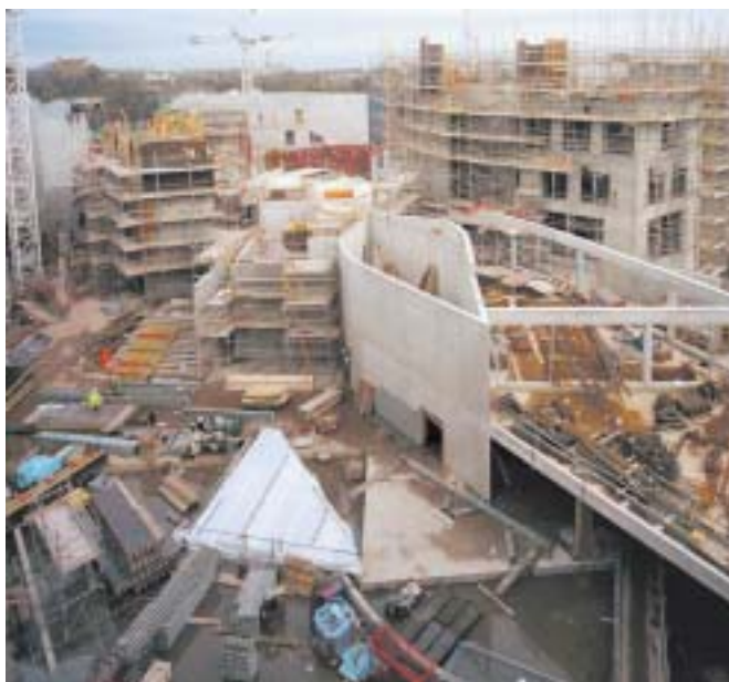
Construction of Committee Towers
