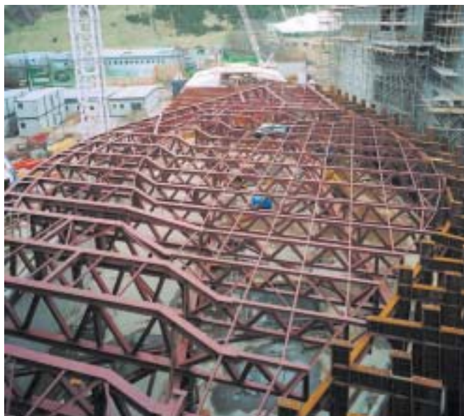
Steelwork on Debating Chamber
