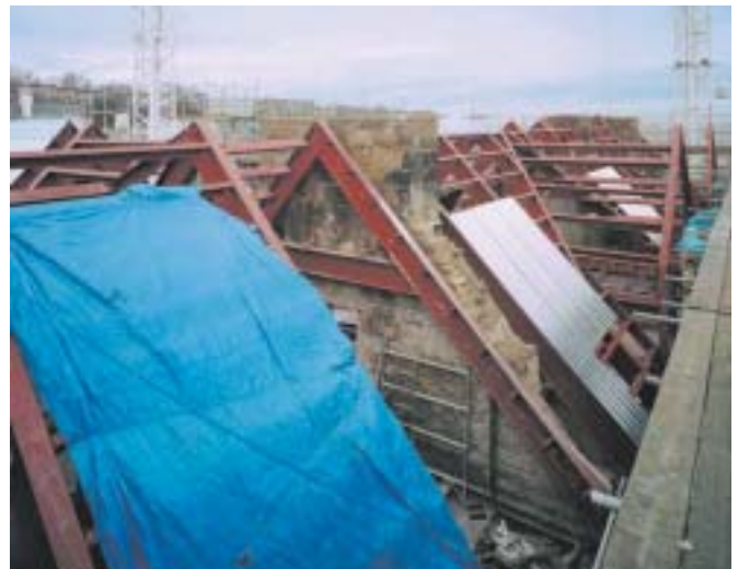
Replacement of Queensberry House roof
