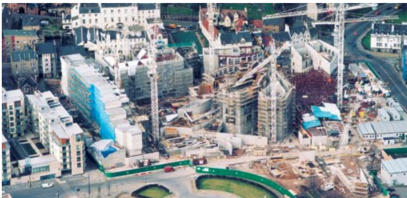
Aerial photo of site
