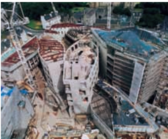
Roofs being installed on the four tower buildings
