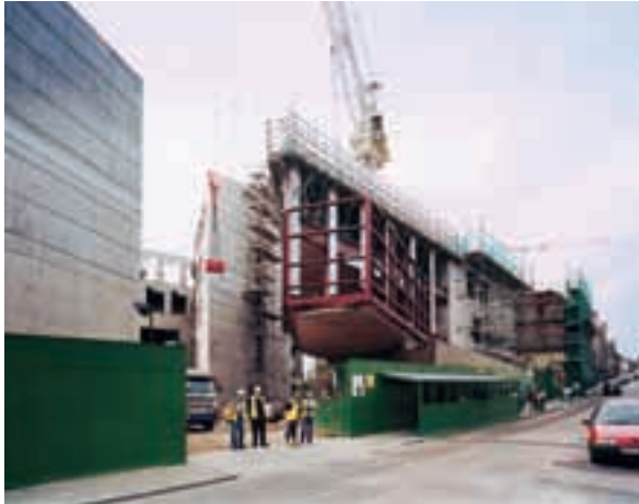
New cantilever building at the foot of the Canongate
