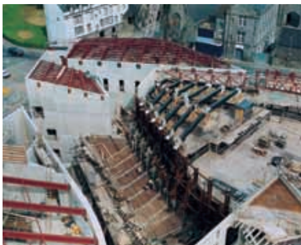
Beams installed on Chamber roof
