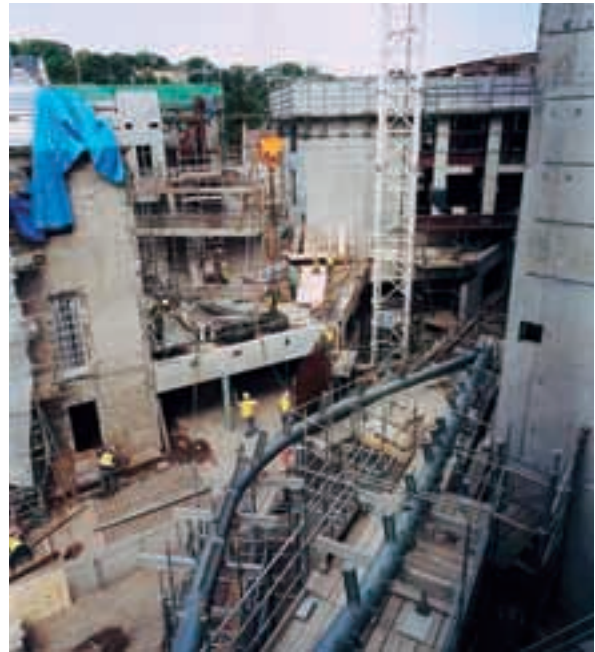
First of the lobby roof lights being installed
