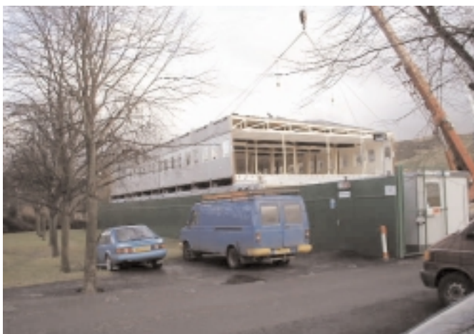
HPT office accommodation under construction February 2000
