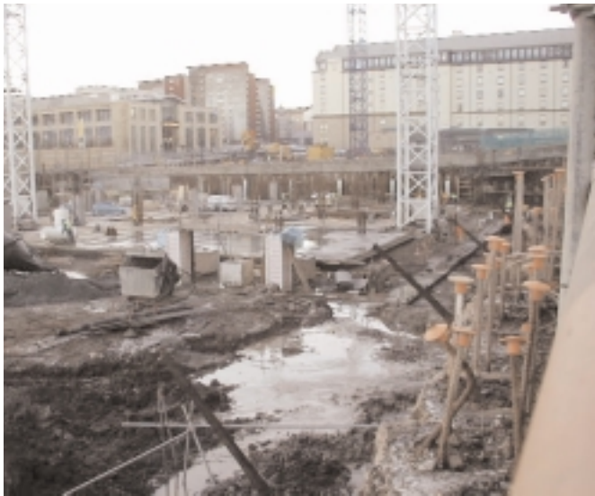
Construction in progress December 1999
