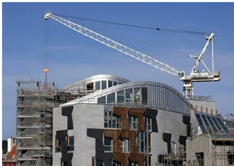
Tower Crane 4 at Holyrood in its final week
