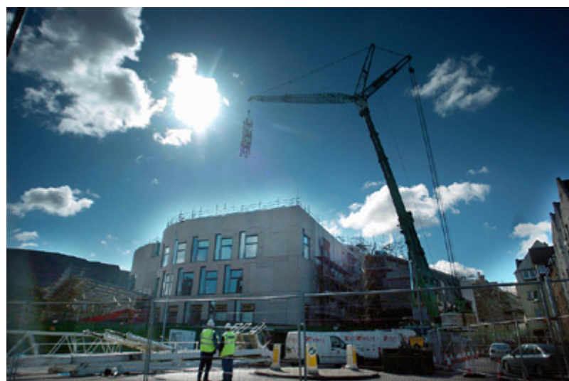
A dismantled Tower Crane 4 leaves Holyrood
