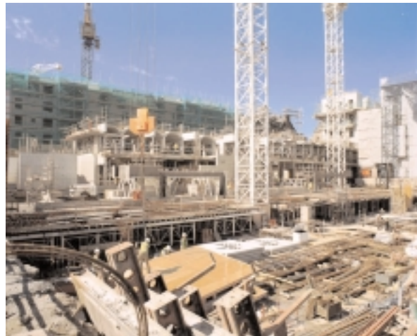
View west across the site - Sept 2000
